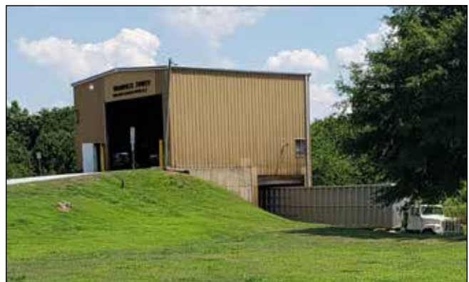
Greenville County's Materials Recovery Facility
